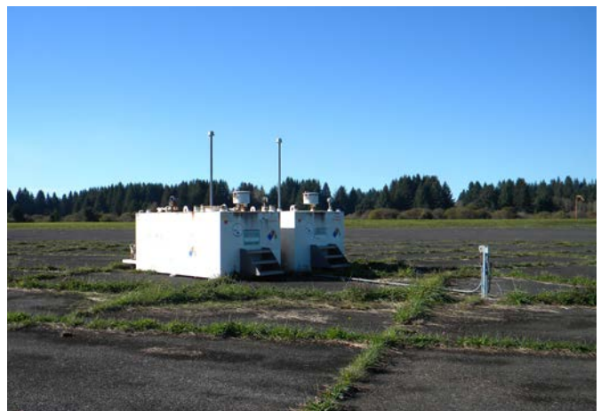
Source: Century West Engineering
