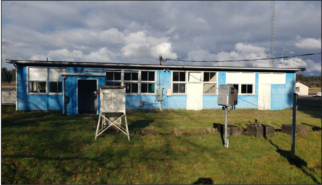
Photo 21. Rear (south) of NOAA building, monitoring instruments in foreground.
