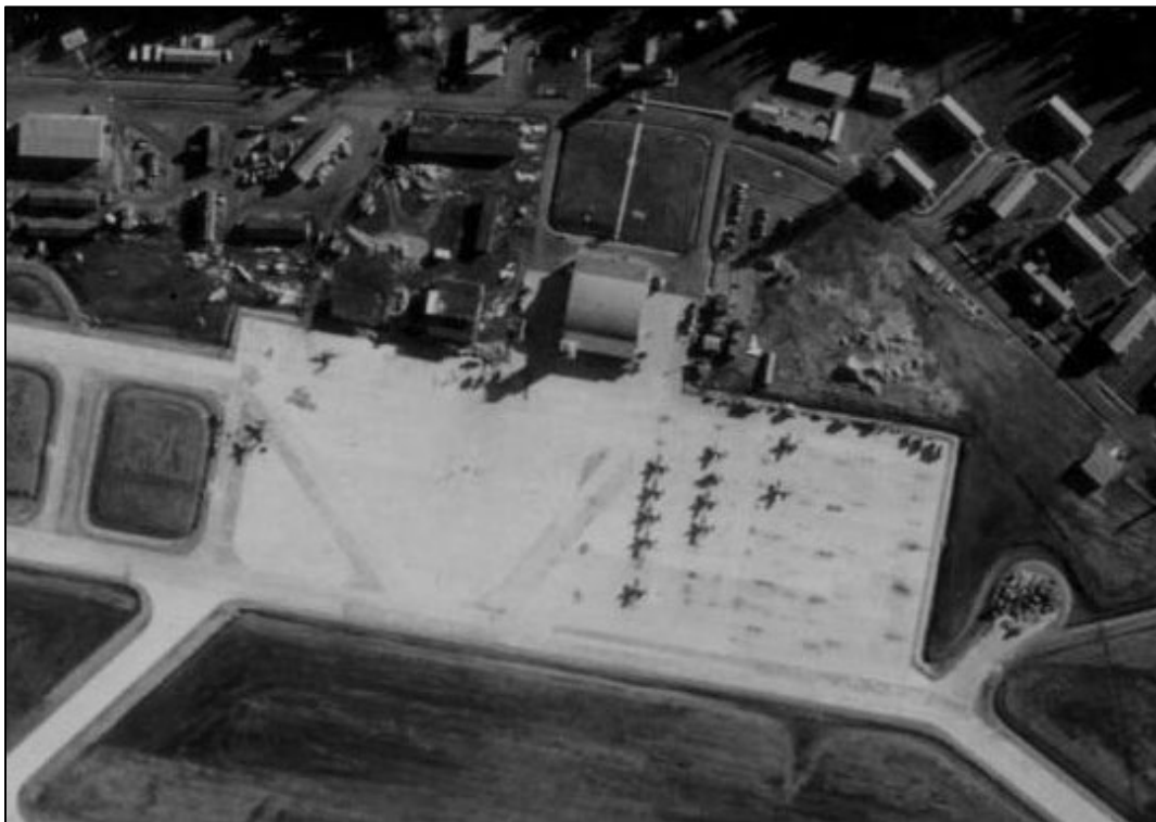
Photo 7. Aerial of hanger and adjoined tower, 1945.
