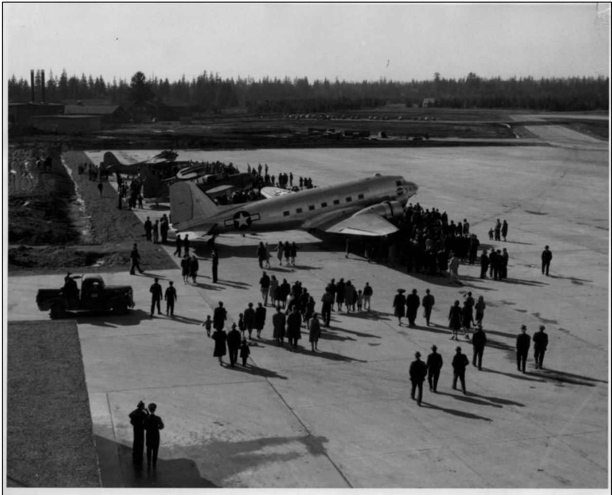
Photo 4. Apron adjacent to existing hanger, date unknown.
