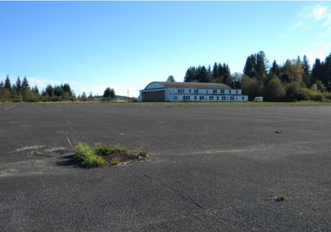
Source: Century West Engineering
