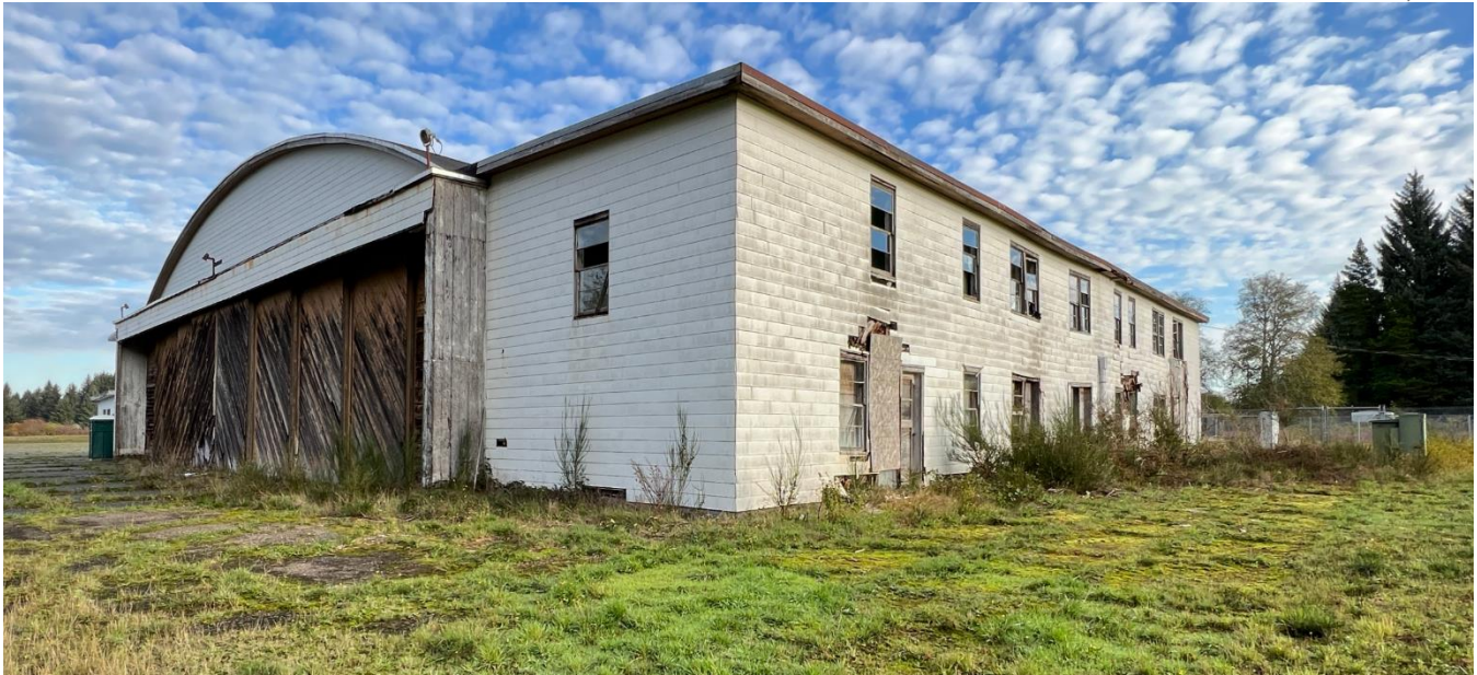
Figure 5: Southwest view of hangar building
