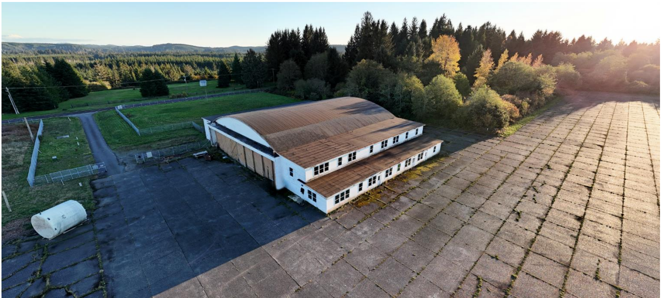
Figure 2: Aerial view of hangar from NE
