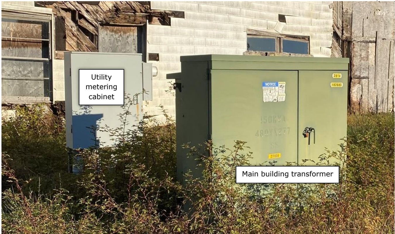
Figure 19: Microgrid PCC location
