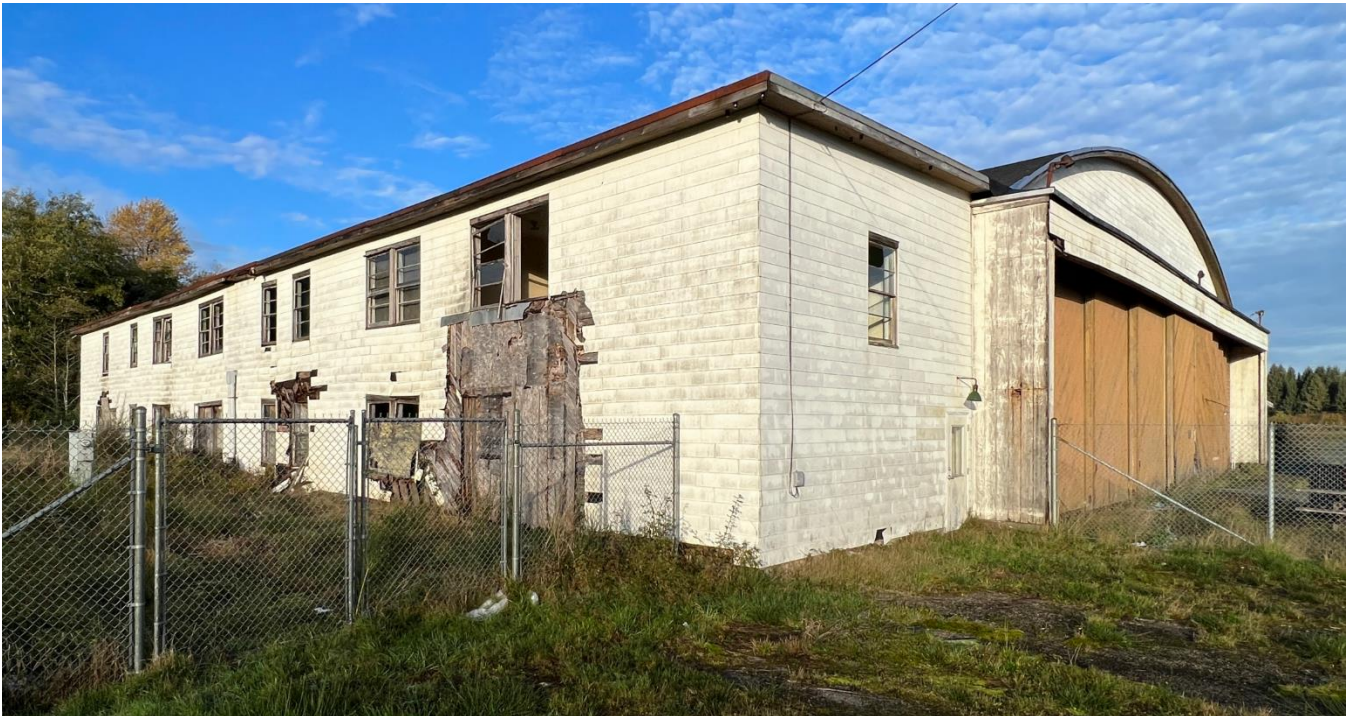
Figure 4: Southeast view of hangar building
