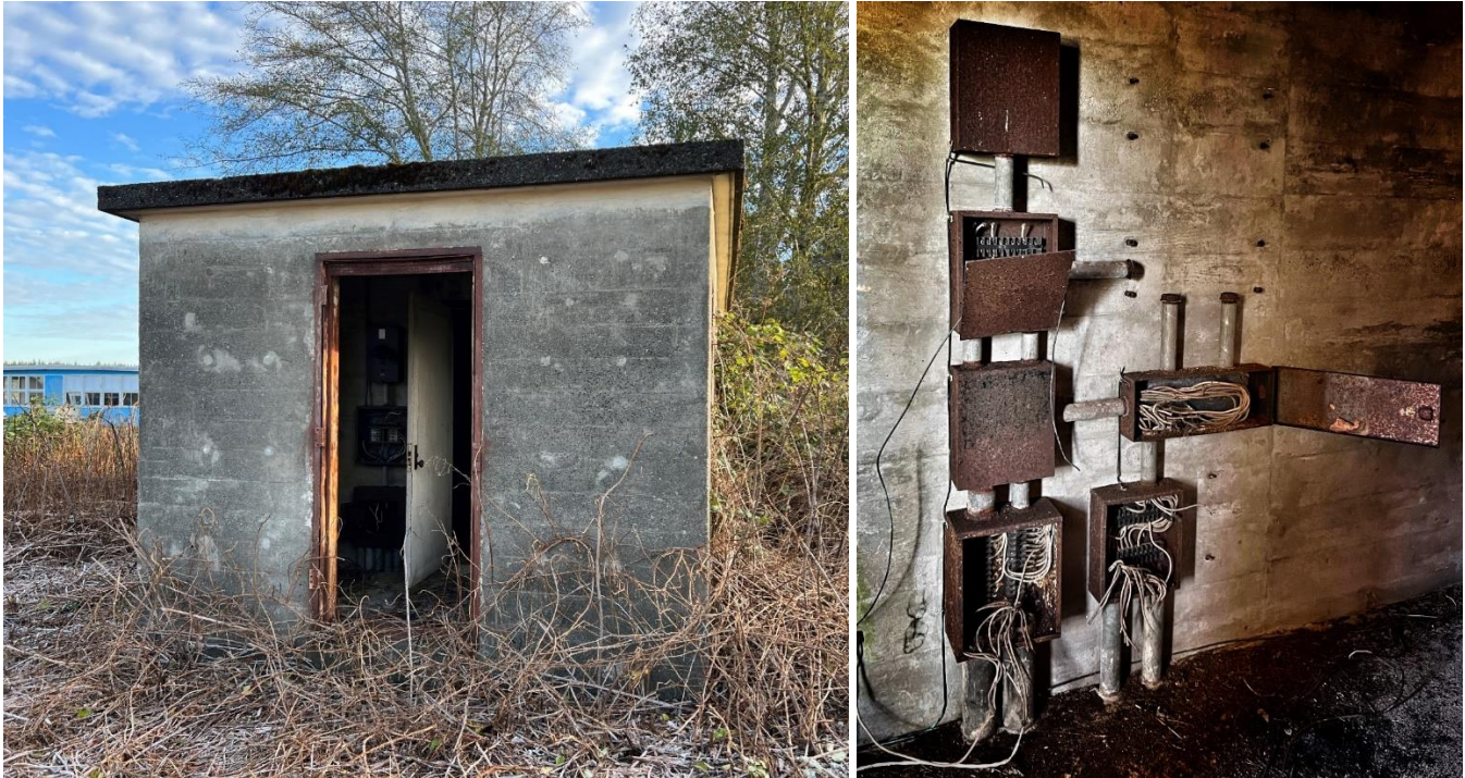
Figure 6: Old power distribution house exterior and interior [left, right, respectively]
